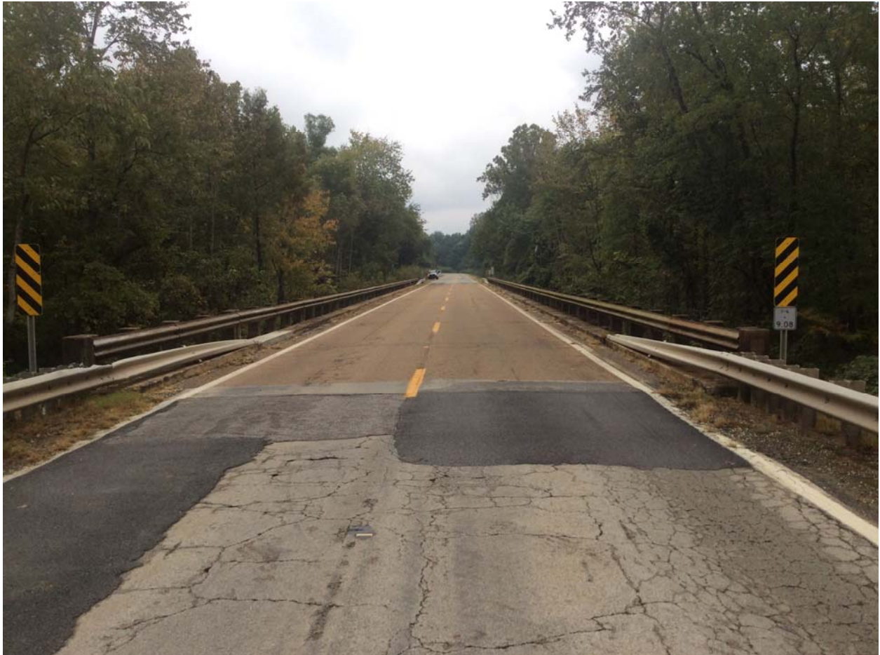
Note: 4" ACHM overlay on bridge deck.
